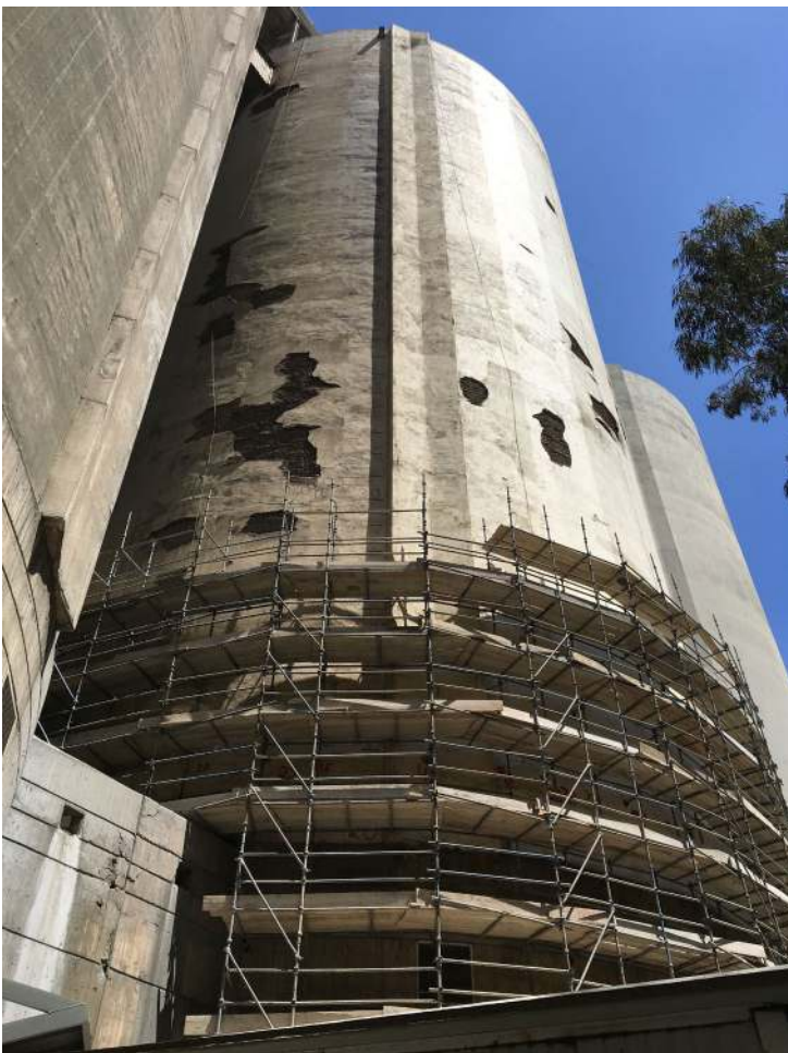
Before remedial works.
